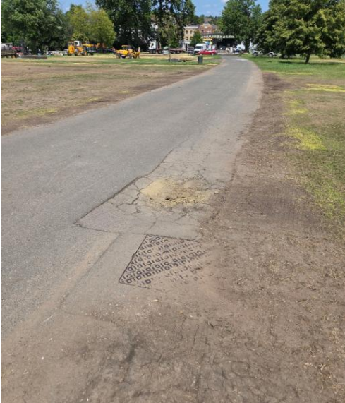
Footpath damage on path from Herne Hill gate to Hall.
