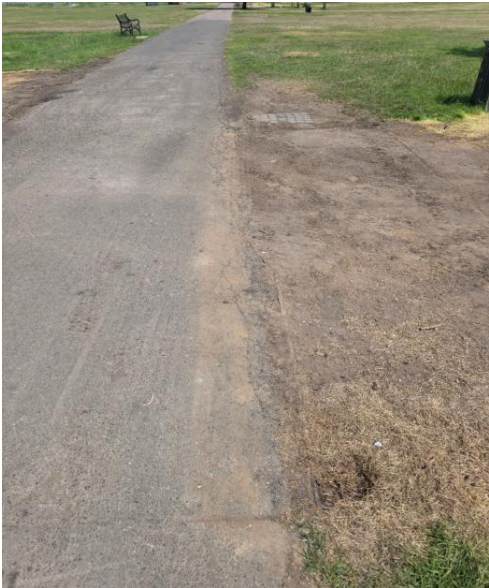
Footpath damage on path from Lido to Tennis Courts.
